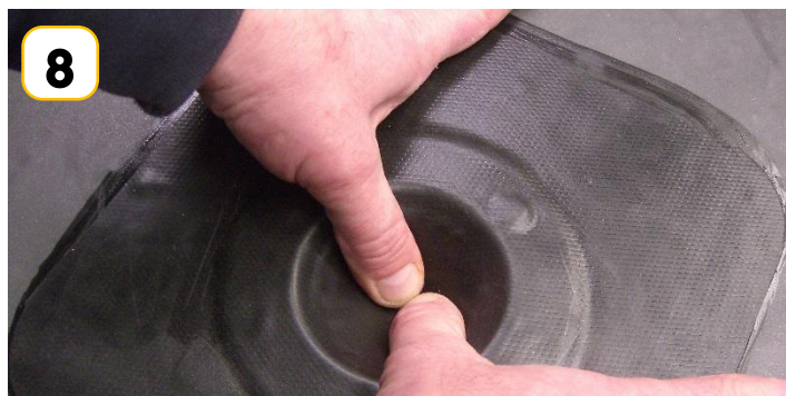
8 Carefully stretch Elasto-form and mould to the inside of the outlet
