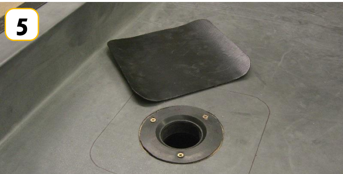
5 Cut Elasto-form patch to size and mark position with pen
