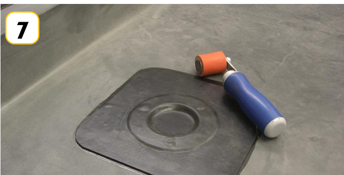
7 Roller Elasto-form tape with seam roller.
