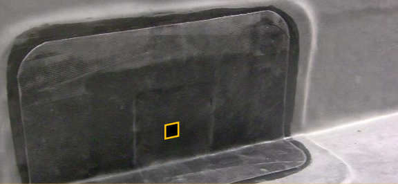
Roller Elasto-form tape with seam roller, & cut small square hole
