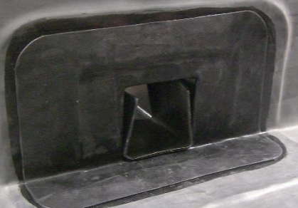
Insert Elasto-form and remove backing film
