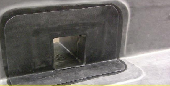
Apply pressure to tape using silicon seam roller
